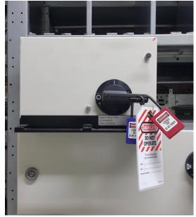
or unexpectedly be powered up or turned on and this would create a hazard, there should be a lockout/tagout procedure to keep the machine safe and guarded while not in use. Compliance with LO/TO procedures prevent hundreds of fatalities and tens of thousands of deaths each year.
