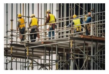
protection below scaffold. Electrocution hazards are principally due to proximity of the scaffold to overhead power lines.
