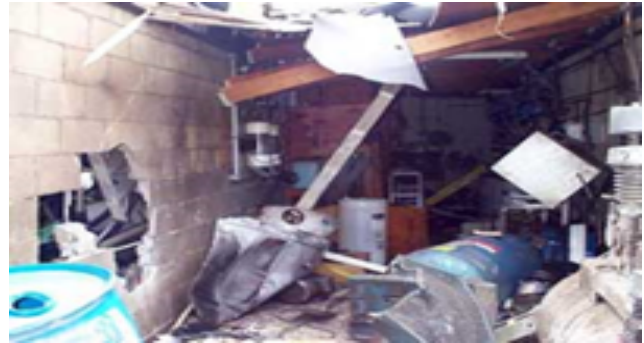
Air Compressor Explosion
