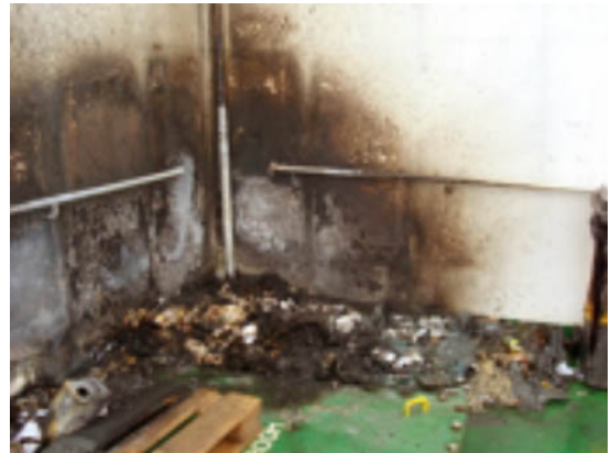
Fire Caused by Spontaneous Ignition (Oily Rags)
