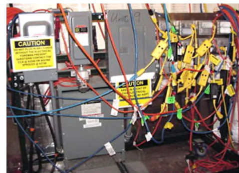
Not the proper use of GFCIs
