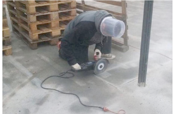
Is this Hazardous?
