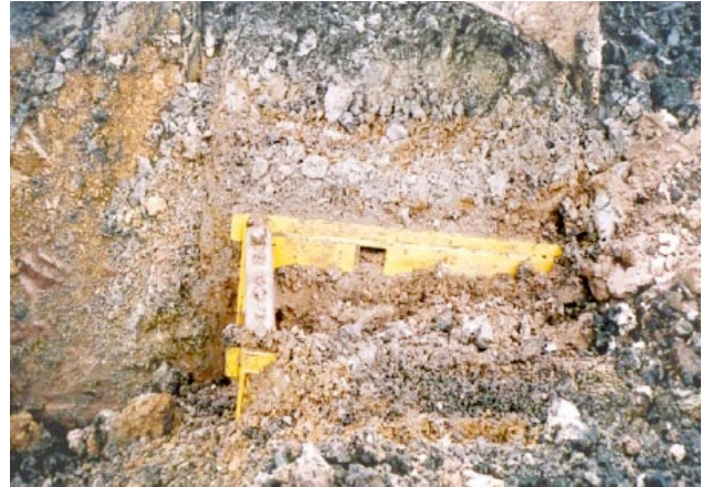
Two workers are killed every month in trench collapses
