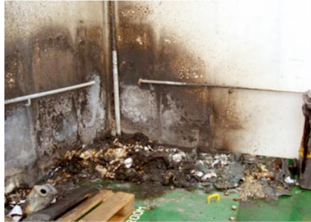
Fire Caused by Spontaneous Ignition (Oily Rags)
