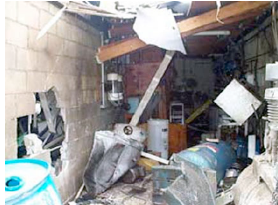
Air Compressor Explosion
