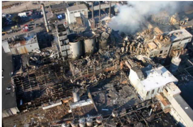
Dust Explosion in Massachusetts
