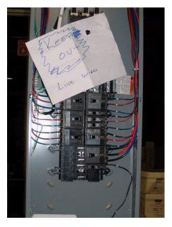
Failure to lock out or tag power sources on equipment can result in electrocutions, amputations, and other serious, sometimes fatal, accidents.
